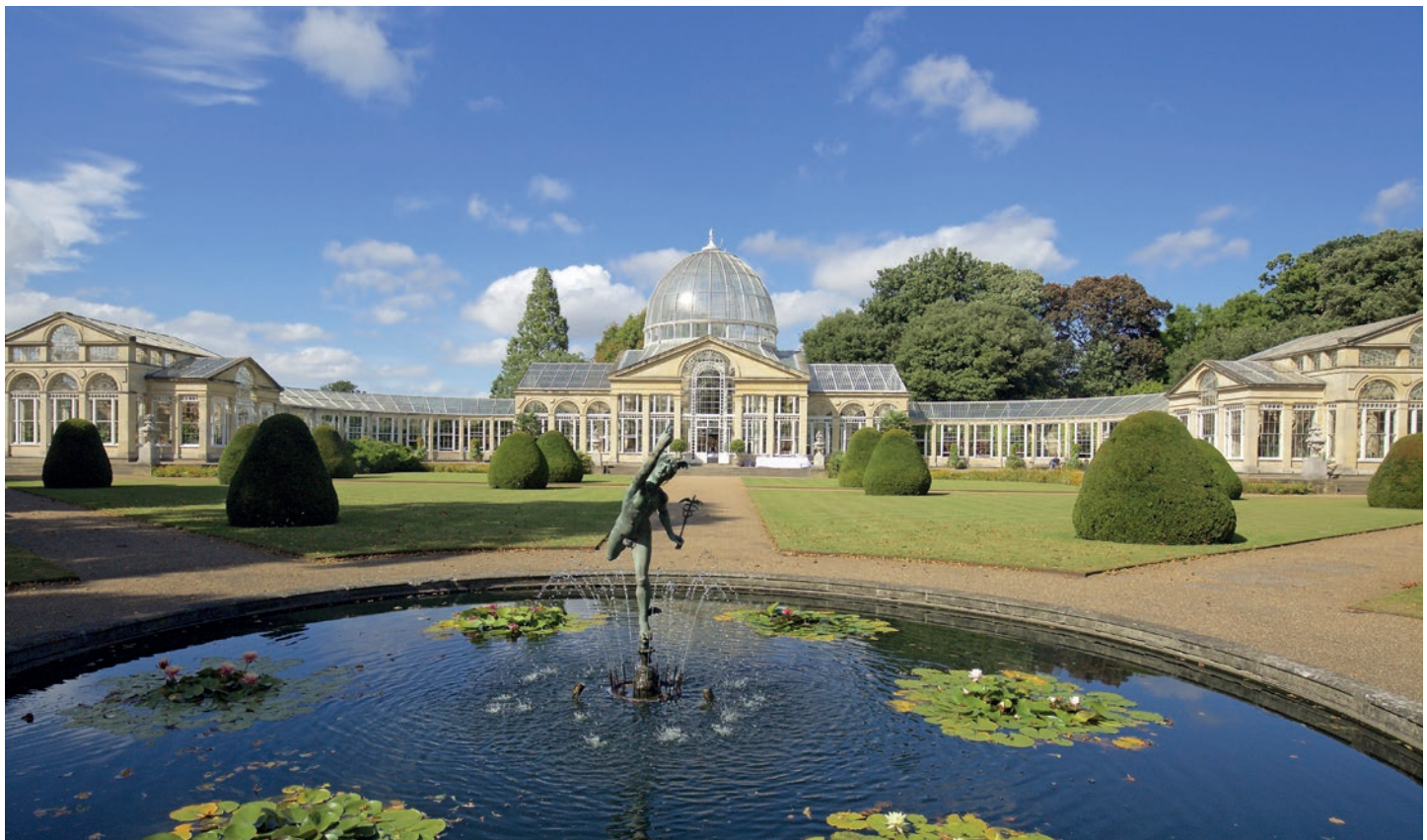
Syon House, London, UK Protected by Advanced MxPro fire panels.
